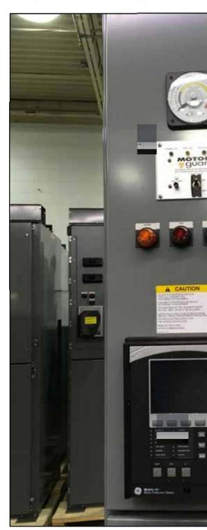
voltage compartment of the MCC or switchgear and directly connects to the motor or generator windings. The unit senses when the motor or generator is offline and then performs a continuous dielectric test on the winding insulation until the equipment is re-started.
