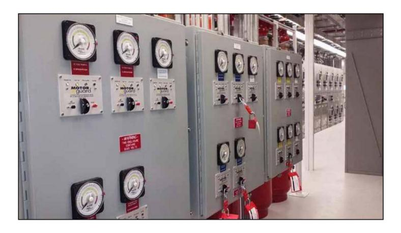
Constant monitoring of critical motors while de-energized prevents failures on startup, reduces unscheduled downtime, saves on major rewinding repairs and increases personnel safety
